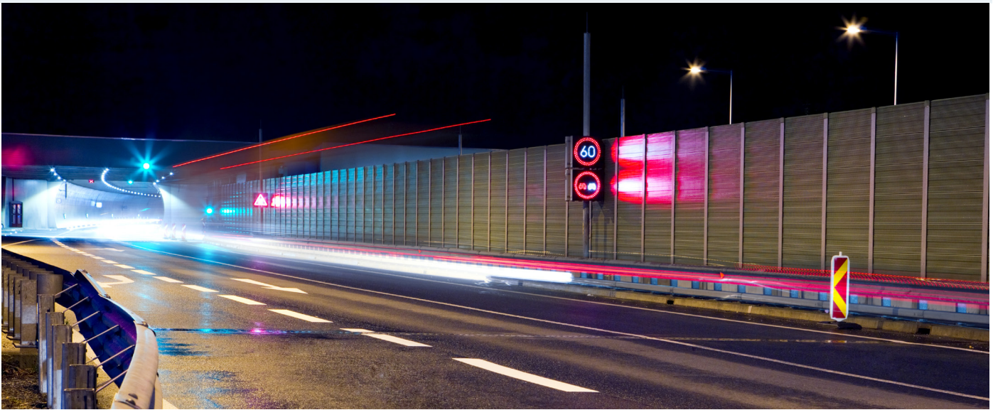
Figure 1: The monitoring system for the Pfänder tunnel is a highly complex application integrating a total of 141 tunnel control units and using 45,000 external system data items.
